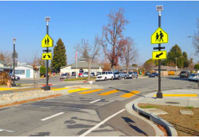
Rapid Rectangular Flashing Beacon (RRFB)
