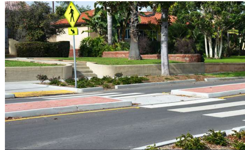
Median Pedestrian Refuge Island
